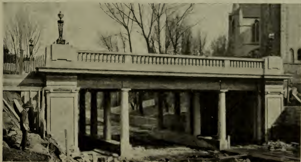
ST. STEPHEN'S ROAD BRIDGE, BOURNEMOUTH, DURING CONSTRUCTION. (See also p. 521.)
